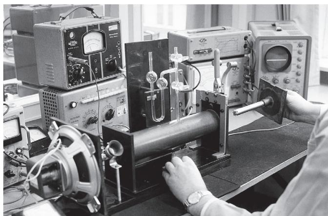
Measuring set-up for the MKH 110 low-frequency microphone
